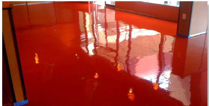
Commercial Restaurant Floor Coated Over Epoxy With X-PROTECT CONCRETE (Clear)
